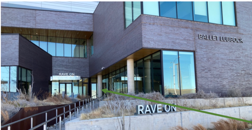
Door to the Right of Rave On
